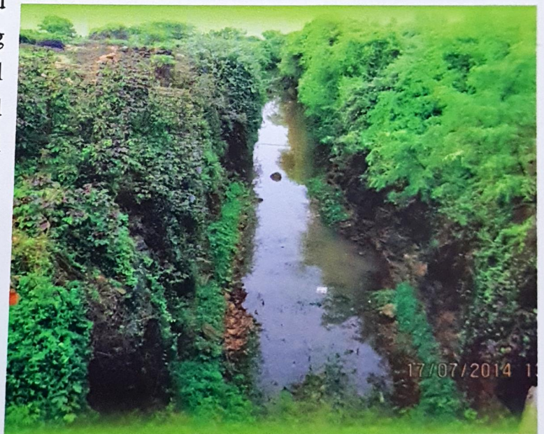
Figure 24: A dugout canal in Mangrol block to connect rivers and rivulets to supply rainwater in coastal areas.
