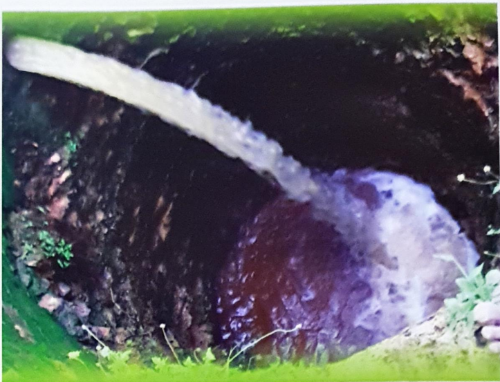
Figure 6: Recharging an open well with runoff water.
